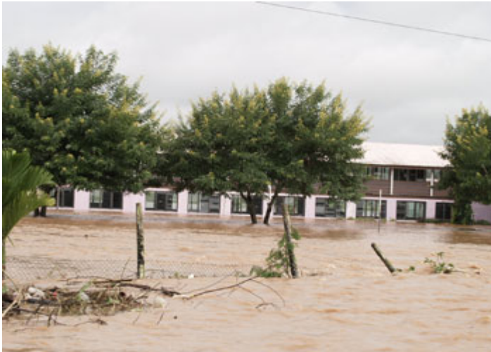
Figure 11. A Navua school partly under water. Source: http://www.fiji.gov.fj/cqi-bin/cms/exec/view.cqi/19/2257
