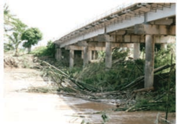
Navua bridge... with debris
