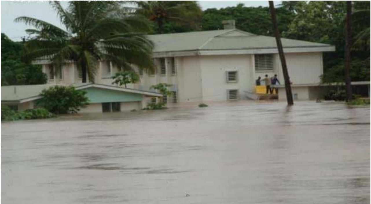
Figure 10. Navua hospital under water, April 2004.
